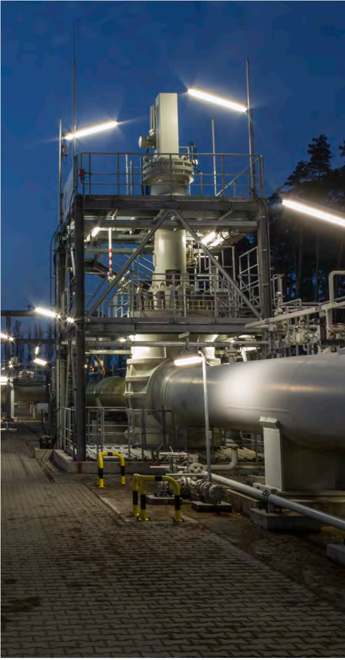
Huge double-gate valves separate the gas in the pipelines from the PIG traps when these are not in operation. They are the heaviest double-gate valves that have ever been produced.
