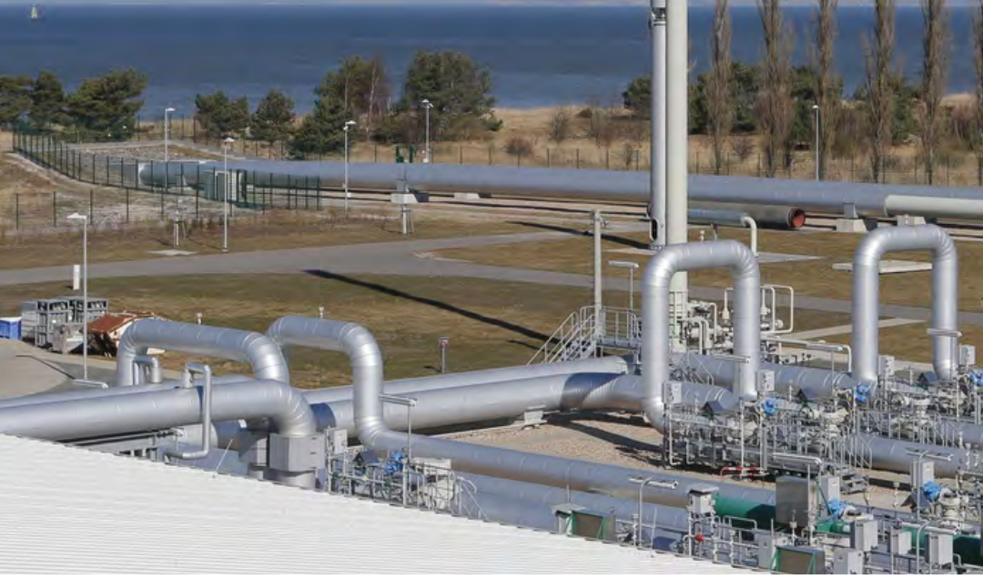
The two lines of the Nord Stream pipeline system reach land at Lubmin. At the landfall station, the natural gas is filtered, measured, and if necessary adjusted prior to transport.
